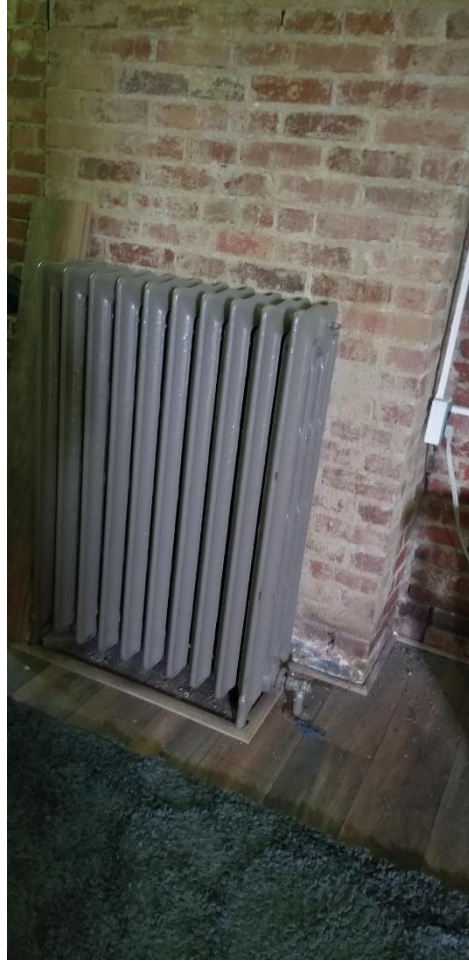
Water heater in officer's room is broken. Firehouse 7
