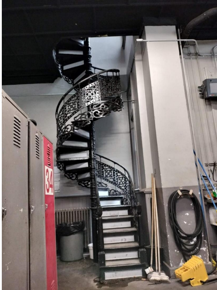
Old style steps from original firehouse design Firehouse 34
