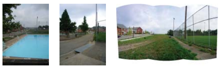
Bedford Hill Housing Development
