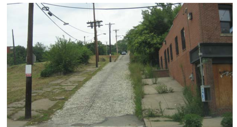
View from Centre Avenue looking at Soho Street
