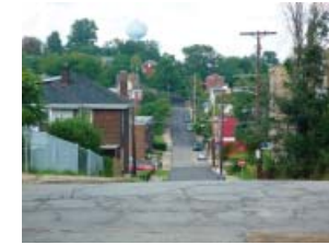
View towards Herron Hill Reservoir
