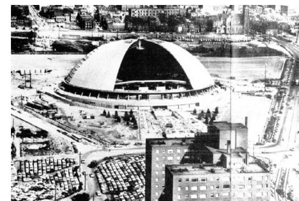
Construction of Mellon Arena, Image from The Lower Hill Renewal and Pittsburgh's Original Cultural District , by William J. Mallett
