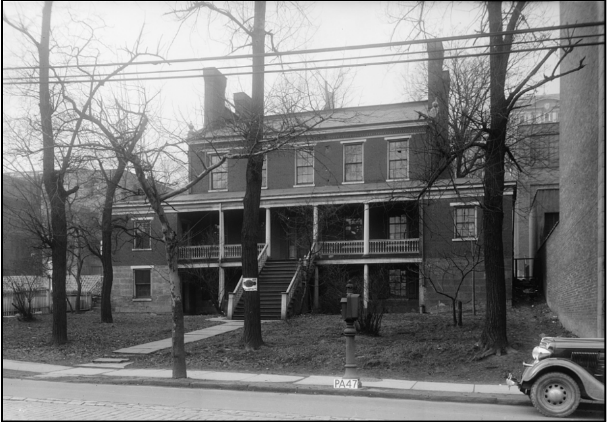
The ca. 1843 Joseph Coltart House, formerly located on Forbes Avenue opposite Coltart Avenue, as it appeared in 1935. Historic American Buildings Survey, Library of Congress.
