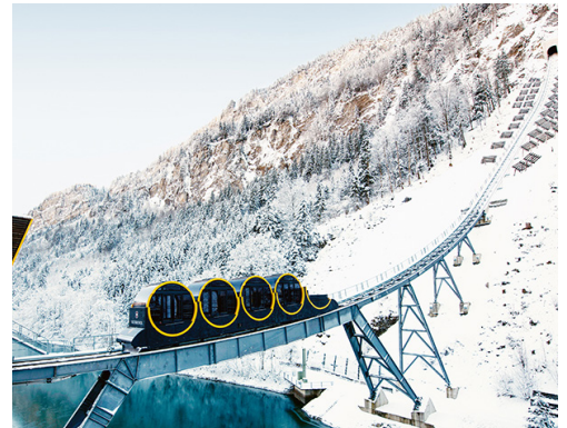
Stoos Funicular is the world's steepest funicular in the world (110%/47.7 degree max incline).
