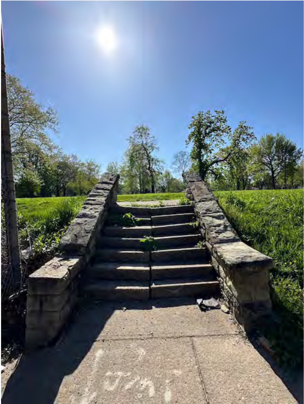
Photo 17. Westinghouse Park, Stairway looking Southeast.
