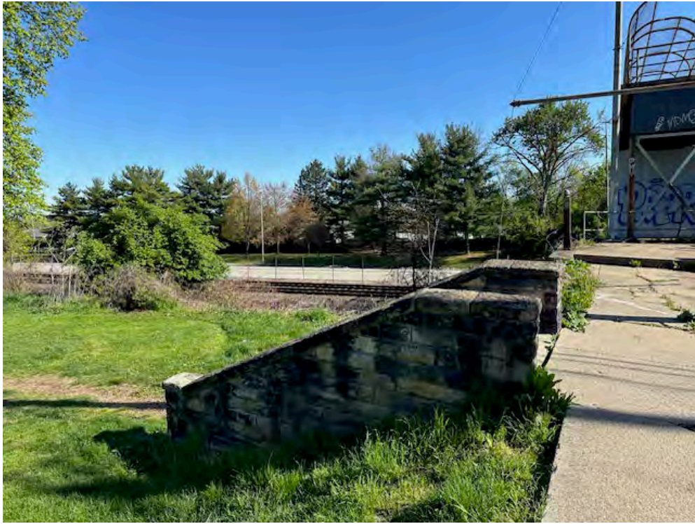
Photo 9. Westinghouse Park, Stone Stairs looking North.
