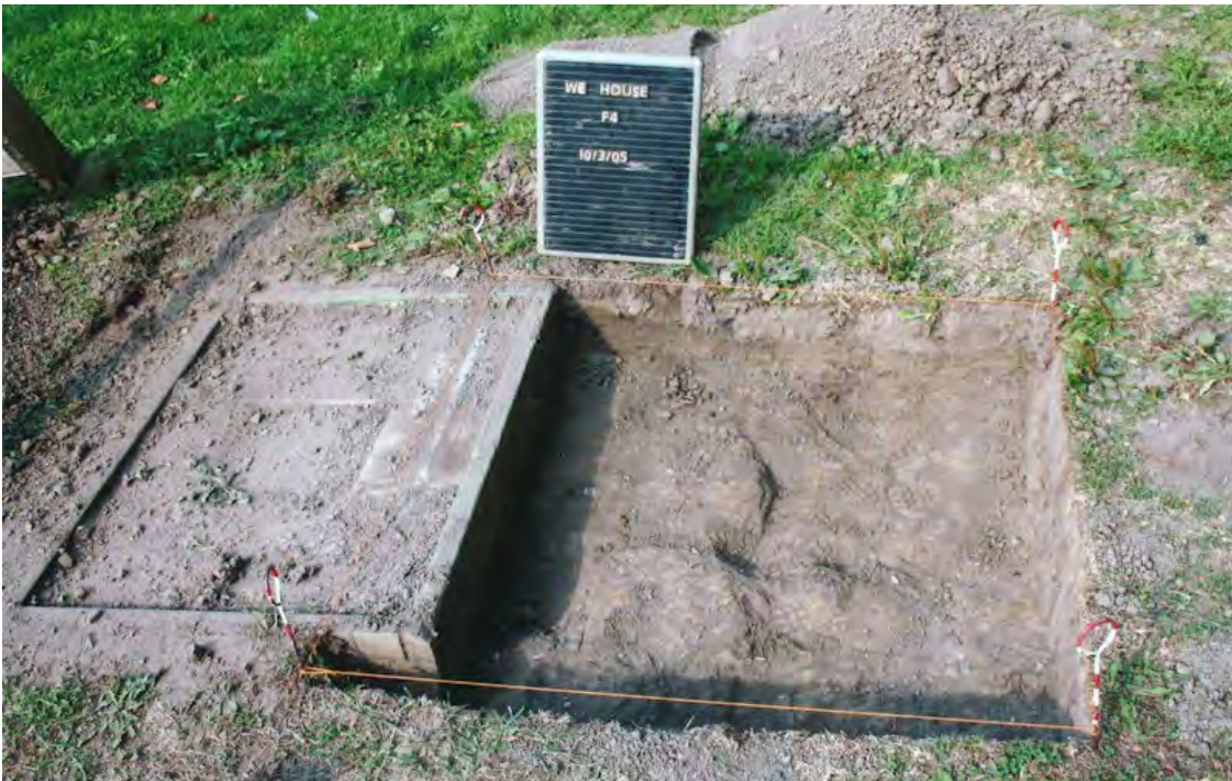
Archeological Photo 14: Feature 4, concrete capped gas well
