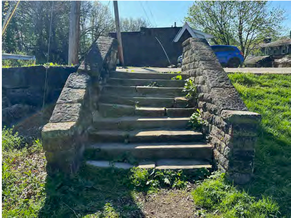
Photo 11. Westinghouse Park, Stairway looking Southeast.
