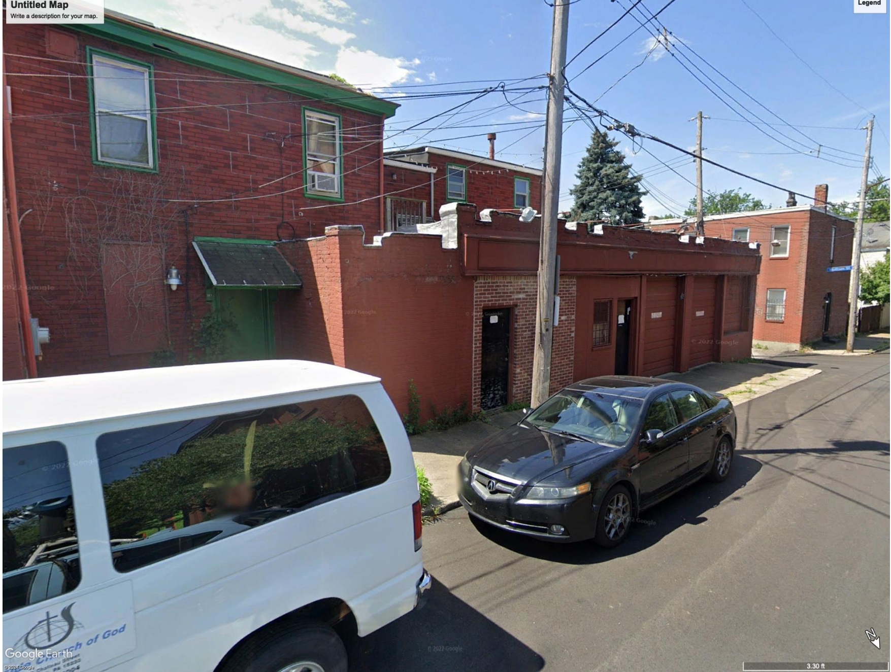
ELEVATION FROM NORTHEAST
