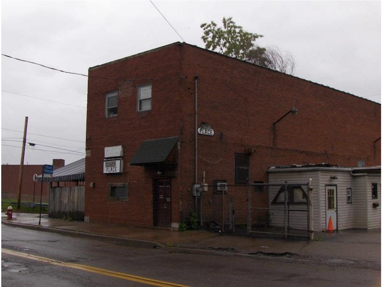
Photo 5 Donny's Place, Primary and western façade, 1226 Herron Avenue. bulldogchicago. Date unknown.
