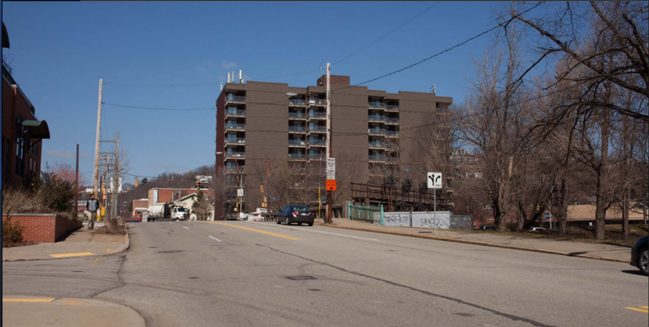
Photo of existing W. North Avenue Bridge from the southwest corner of Brighton Road and Beech Avenue, facing north.
