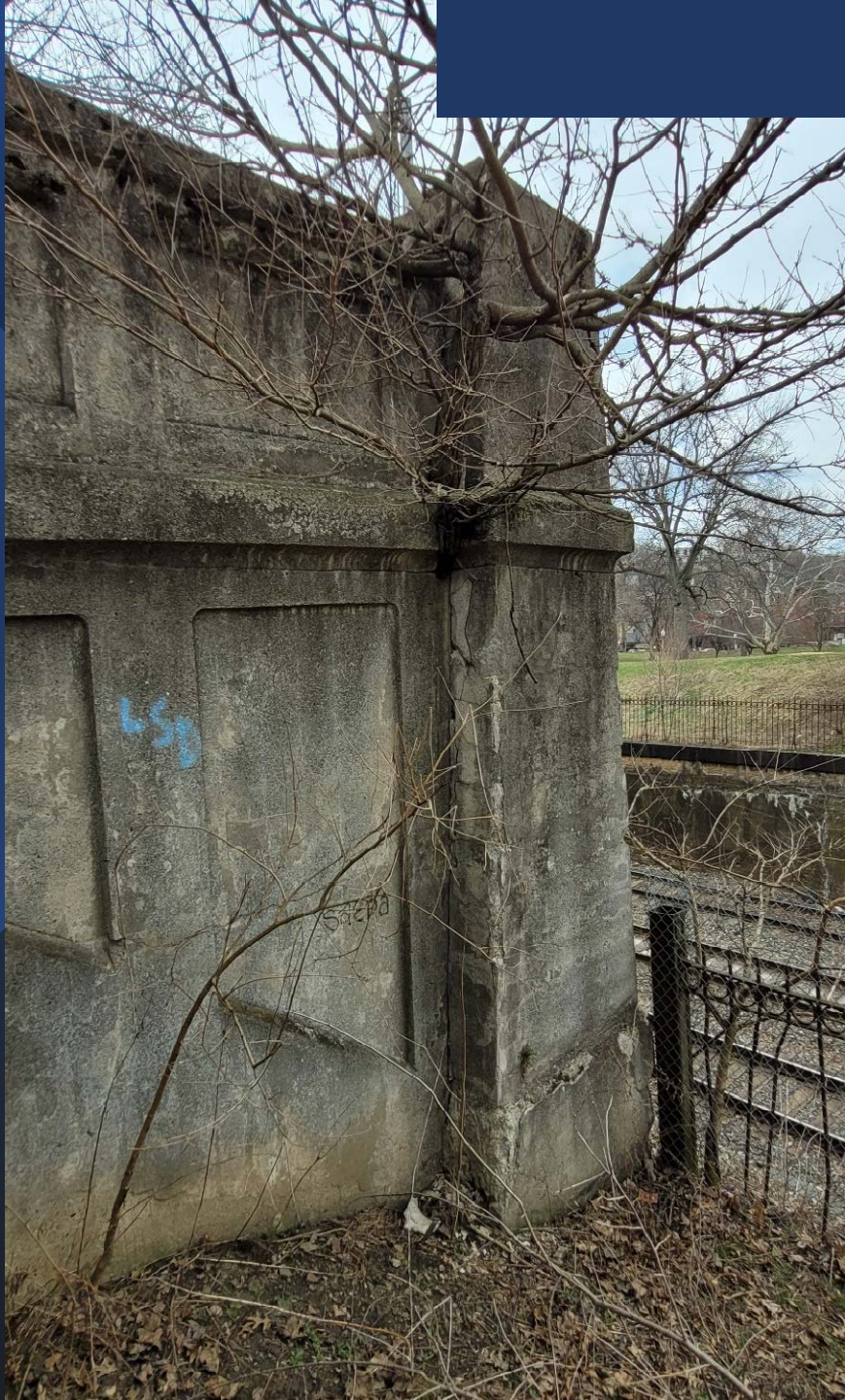
Detail of concrete panels on existing pedestrian bridge abutments.
