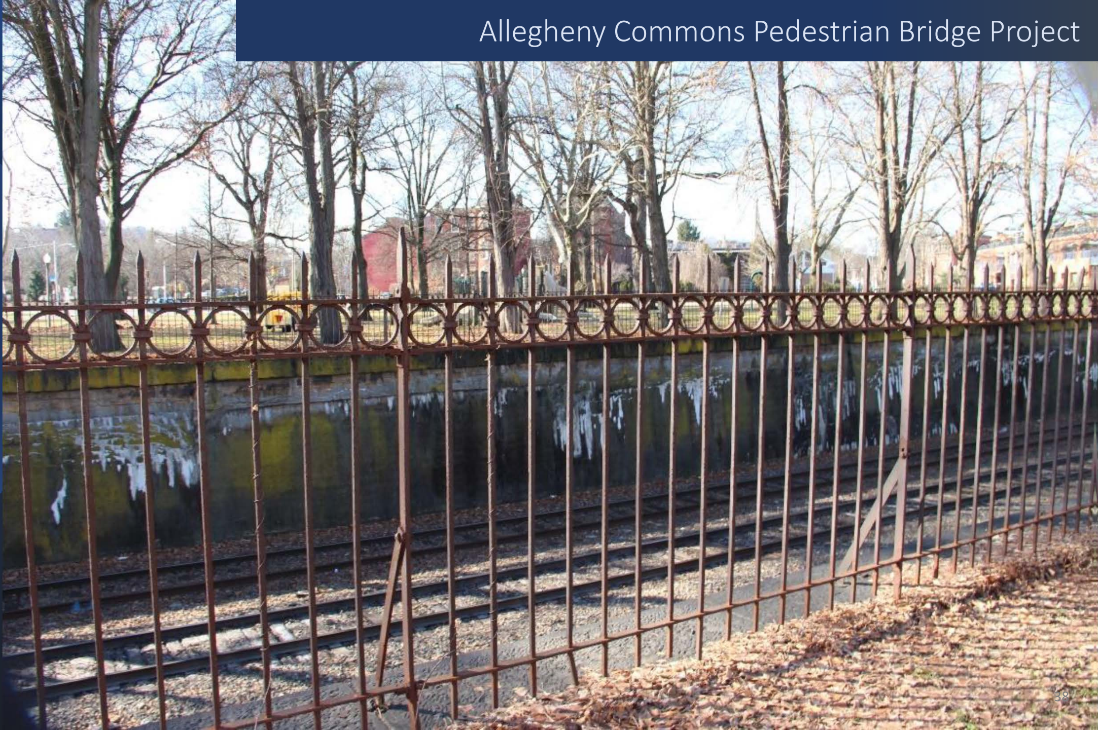
Detail of wrought-iron fencing atop retaining wall, facing southwest.
