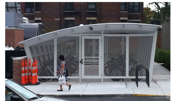
Example of Secure Bicycle Parking - MIT Campus, Cambridge
