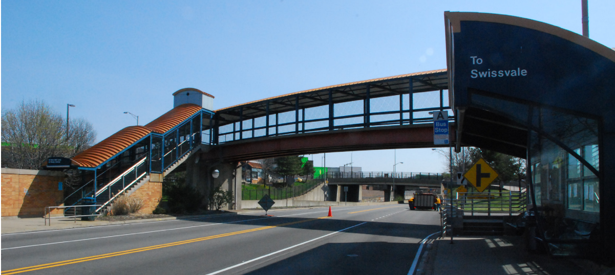
Looking west from the station platform
