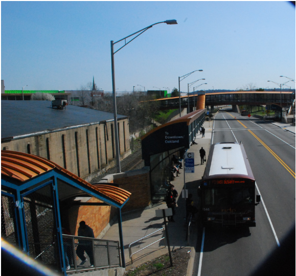
The station from the western pedestrian bridge
