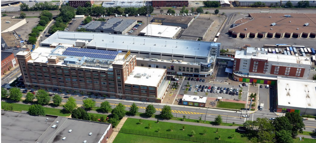
Bakery Square - Photo: Pittsburgh Urban Redevelopment Authority
