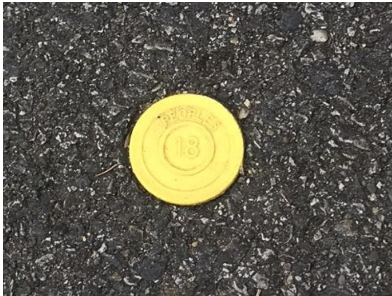
Peoples Natural Gas tag, installed 2018
