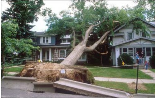
USDA Forest Service photo of curb and house damage from an uprooted tree.
